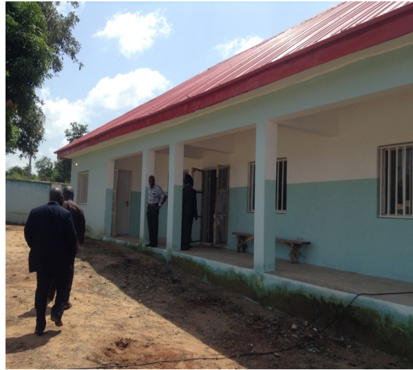
Constructed Maternal and Child Health care centre
